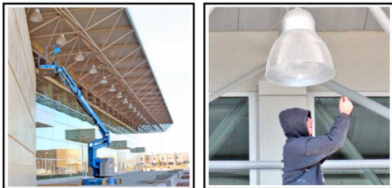
TRICON expertly installed more than 25,000 sq ft of K-net
