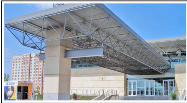
The open frame design was an open invitation to pest birds.
